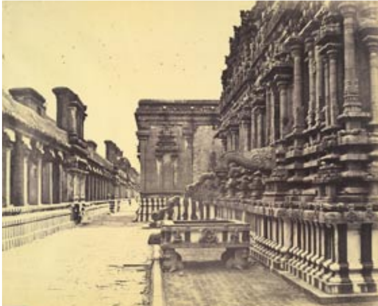
FIG. 11 Captain Linnaeus Tripe Sacred cistern and water spout belonging to the Subrahmanya Swami's Temple 1858
